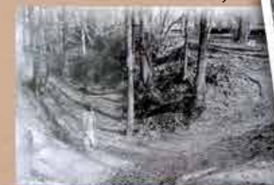
Perimeter Ditch, circa 1947, courtesy Athens-Limestone Historical Society.
