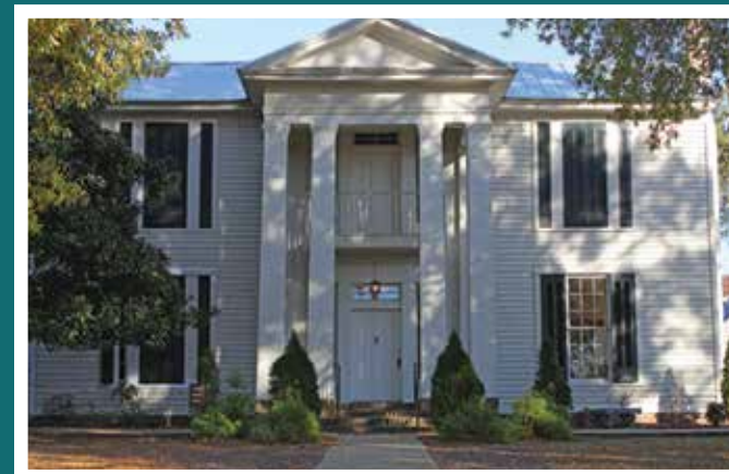
STOP 1 DONNELL HOME "PLEASANT HILL" CA. 1851 601 SOUTH CLINTON STREET
