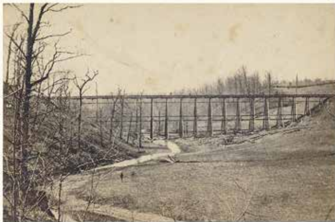
Sulphur Creek Trestle, 1864.
